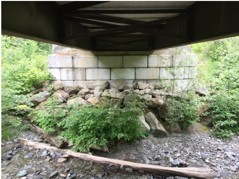
Left Bank Abutment when facing downstream
