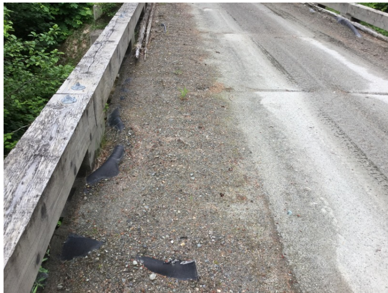
Rubber mats along both edges of deck
