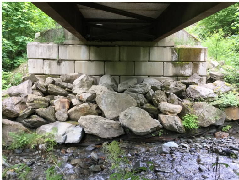
Right Bank Abutment when facing downstream
